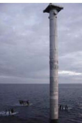
... and almost successfully installed
