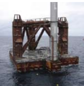
Yme substructure installation, ballasting
