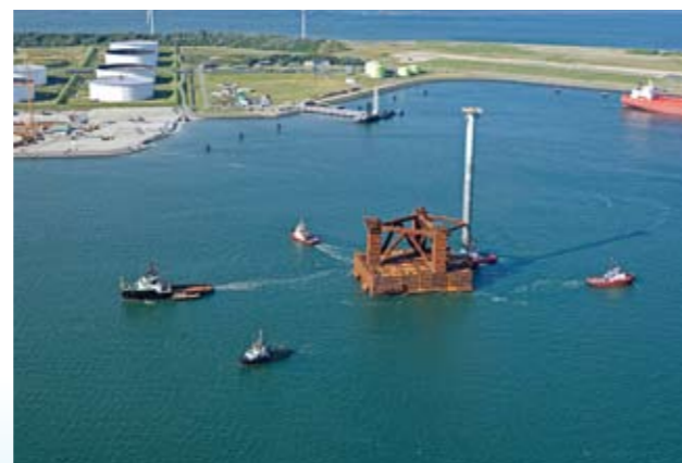
Yme MOPUstor subsea storage tank - under tow in Rotterdam - Beerkanaal, Maasvlakte
