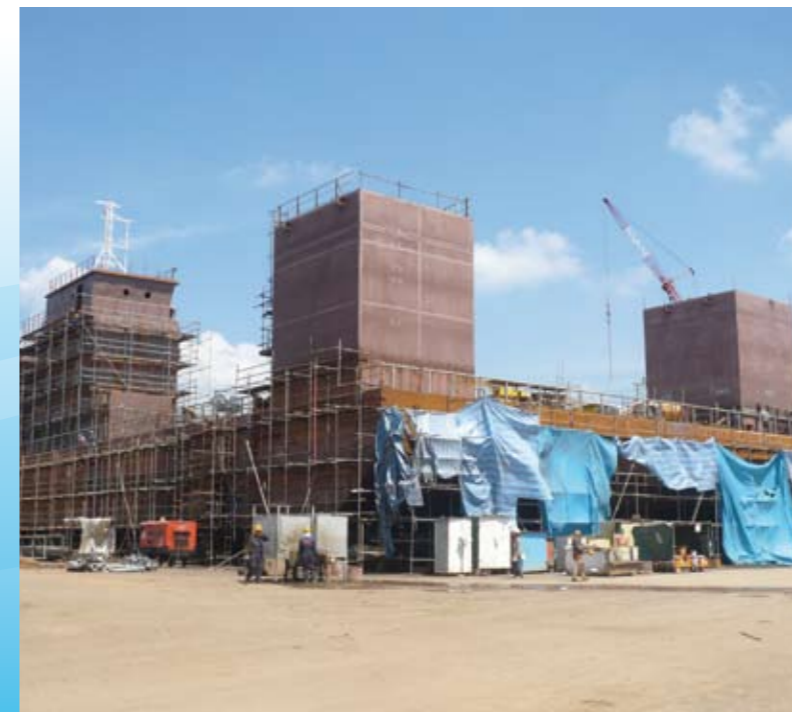
JB-114 under construction
