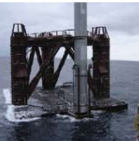
Yme substructure installation, ballasting
